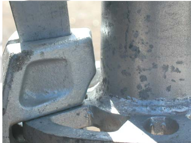
Crack in rosette, test #2 at 11,500 lbs.
